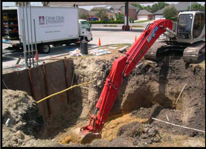
UST Removal and Subsurface Sampling
