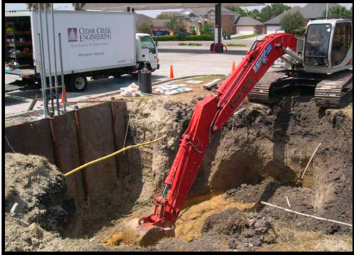
UST Removal and Subsurface Sampling
